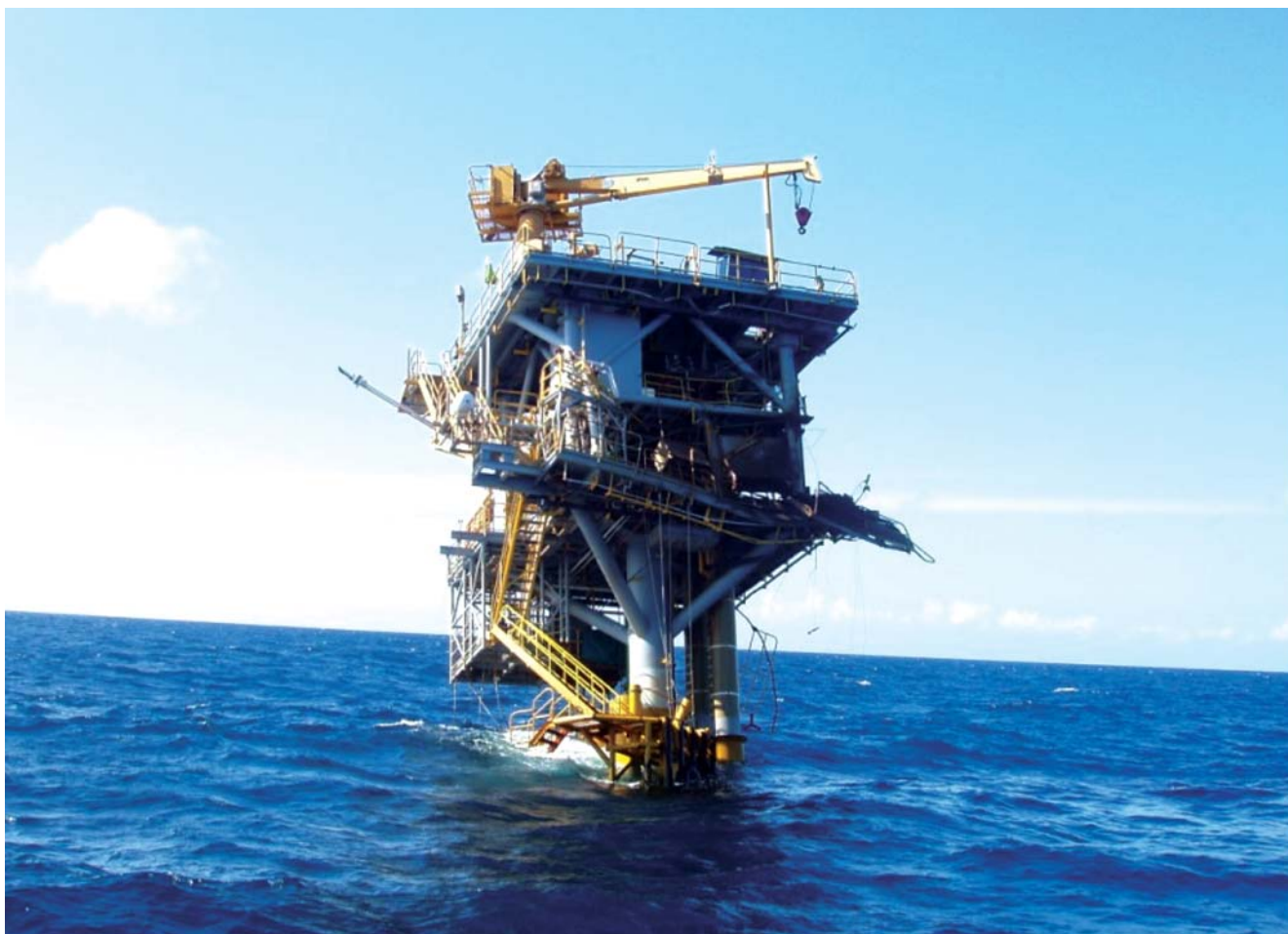
A platform in Indonesia that collapsed due to a ship collision [1]
